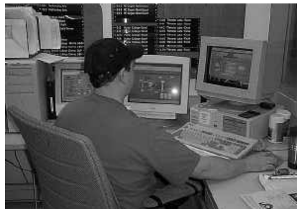
Cogen Plant Watchstander being attentive to the energy management system computers.
